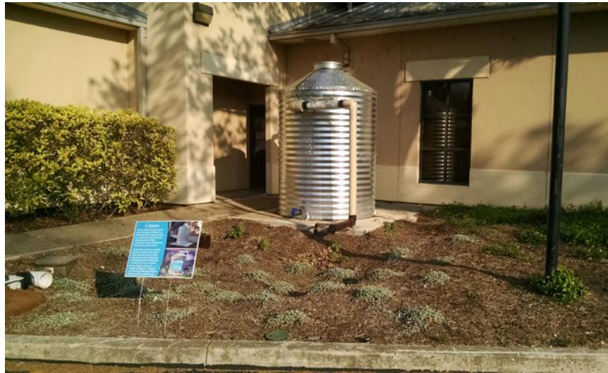
Figure 2-17: Example of a roof leader cistern
