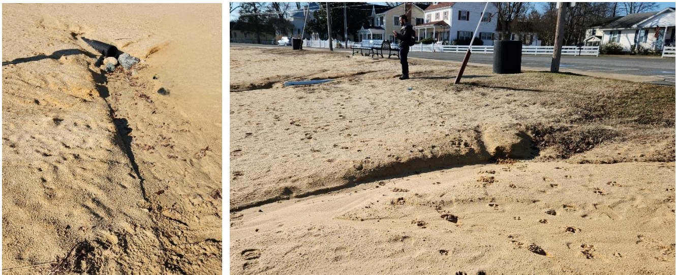
Figure 2-11: Beach scouring at an outfall (left) and from pavement (right) along Beach Terrace/Irving Avenue (February 1, 2024)
