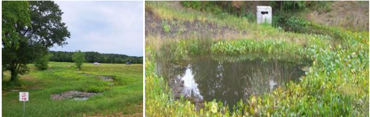
Figure 2-9: Examples of a constructed submerged gravel wetland (left) and a stormwater BMP constructed wetland pond (right) planted with native non-invasive plants
