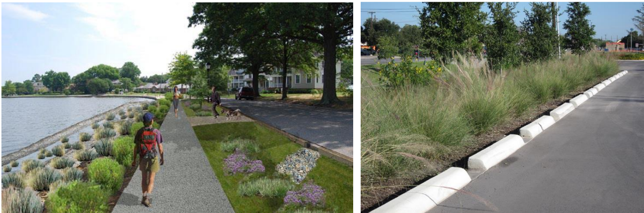
Figure 2-10: Green stormwater infrastructure, vegetated dunes, and bioswale examples
