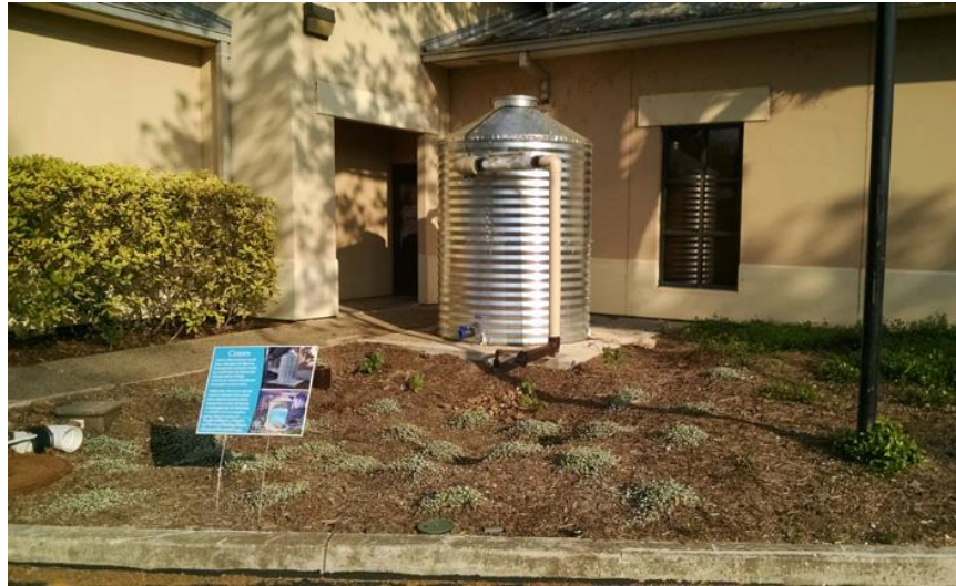
Figure 2-13: Example of a roof leader cistern
