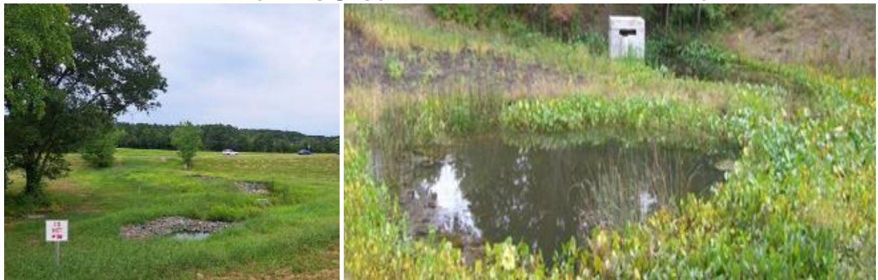
Figure 2-8: Examples of a constructed submerged gravel wetland (left) and a stormwater BMP constructed wetland pond (right) planted with native non-invasive plants
