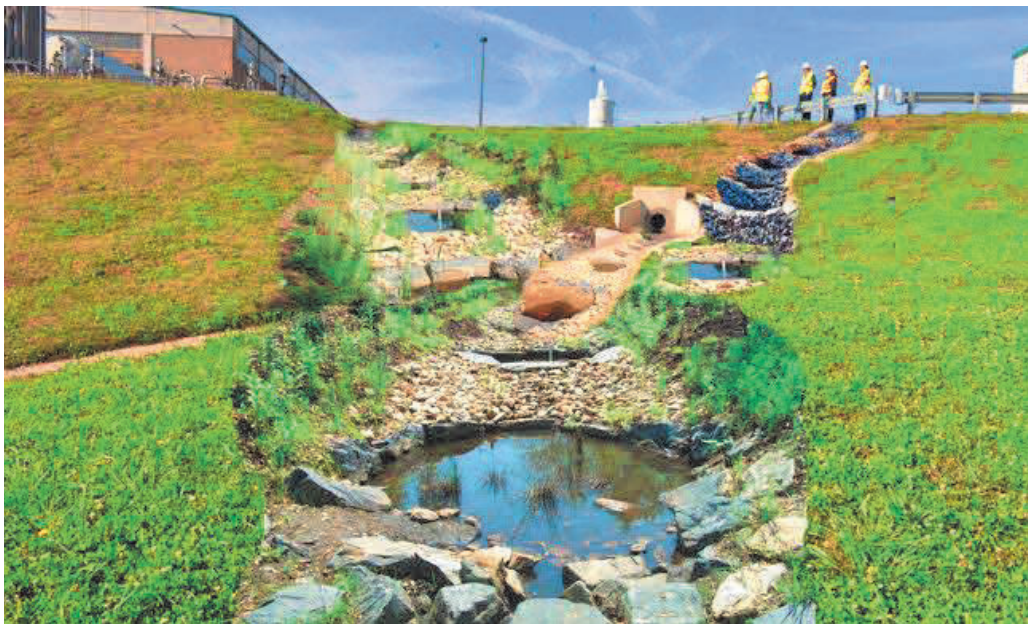
Figure 2-9: Stormwater outlet end treatment example: Regenerative stormwater control (RSC) measures
