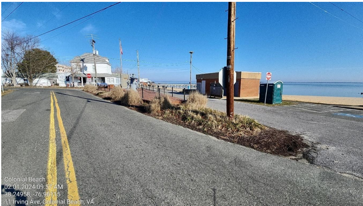
Figure 2-18: Opportunity for small bioretention swales along the sides of the Cannon War Memorial and a bioretention pond/rain garden at the Point (February 1, 2024)
