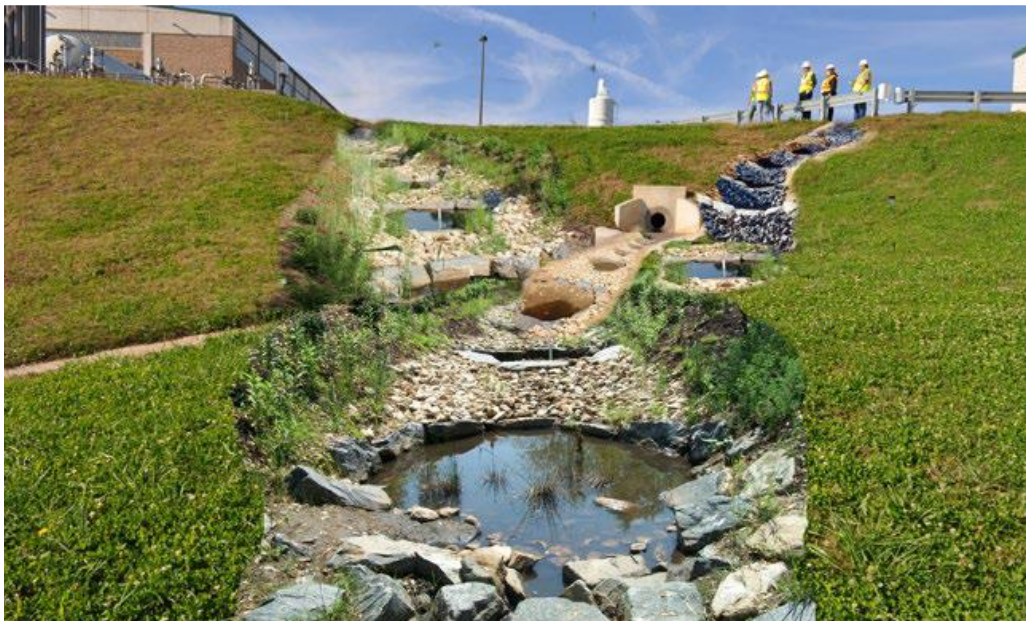
Figure 2-13: Stormwater outlet end treatment example: Regenerative stormwater control (RSC) measures
