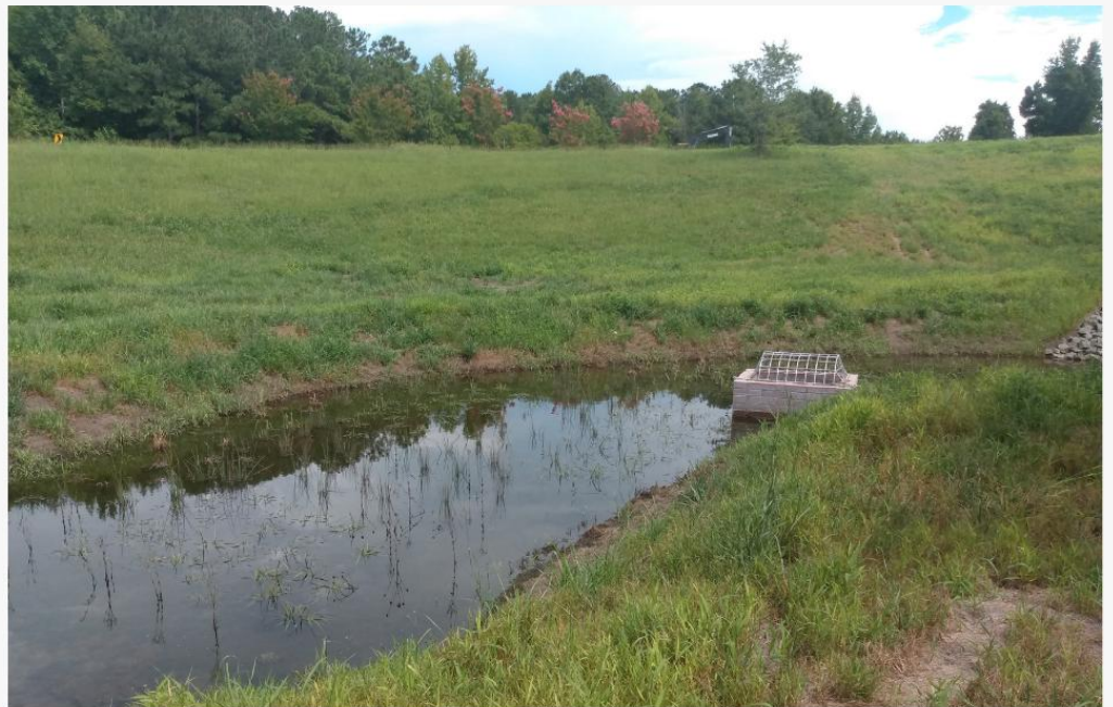
Example of constructed wetland
