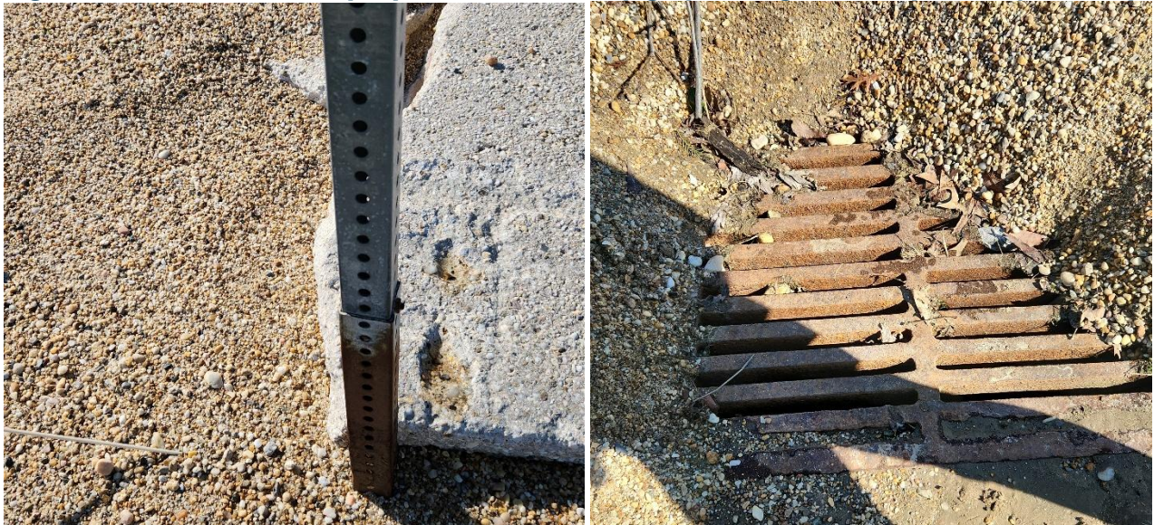
Figure 2-20: Buried Outfall (left) and Buried Inlet (right) on Virginia Ave (February 1, 2024)
