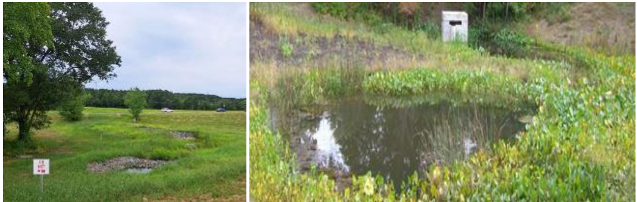
Figure 2-9: Examples of a constructed submerged gravel wetland (left) and a stormwater BMP constructed wetland pond (right) planted with native non-invasive plants
