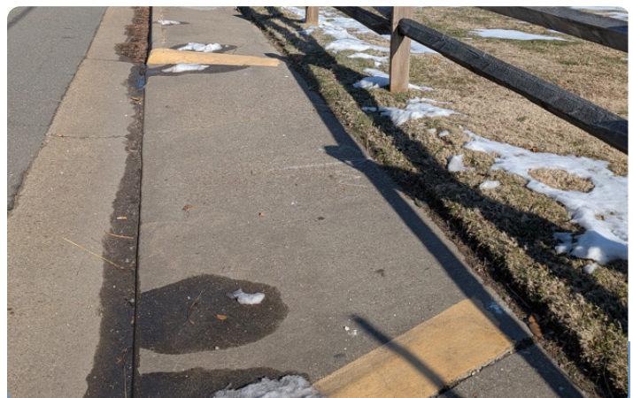
Curb cut not used as a driveway
