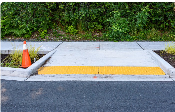
ADA-compliant curb ramp
